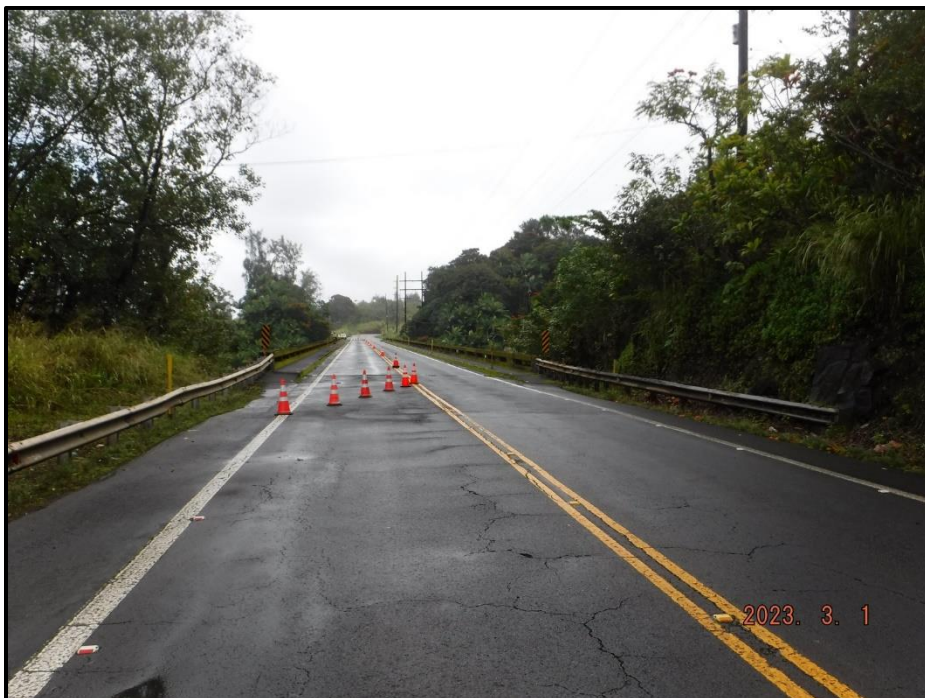
Photograph 4. North approach, looking south.
