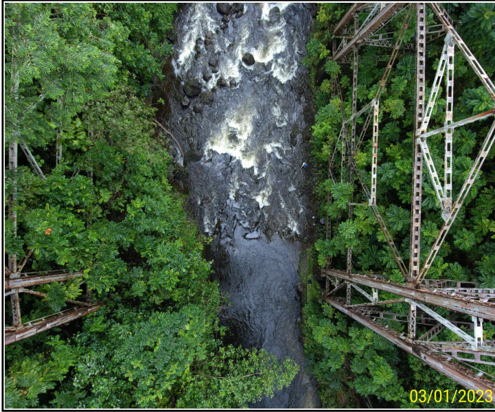
Photo 5. Typical channel overview
