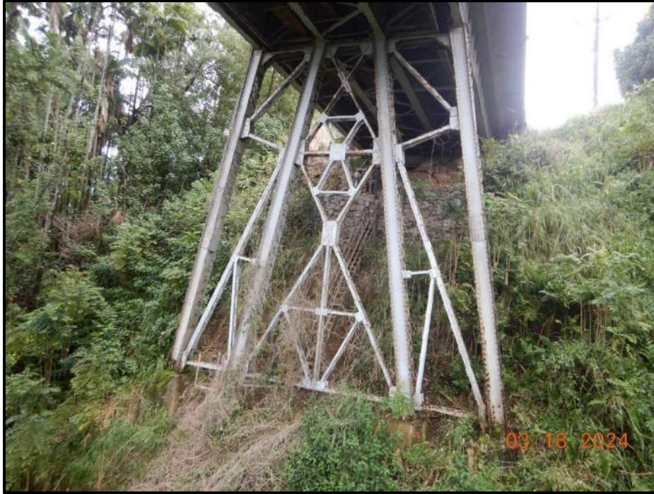
Photograph 7. Bent 1 at Tower 1 (north face shown), looking south.
