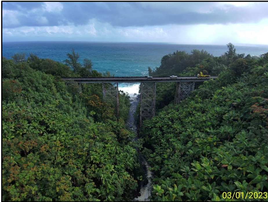
Photograph 1. West (upstream) elevation, looking east.
