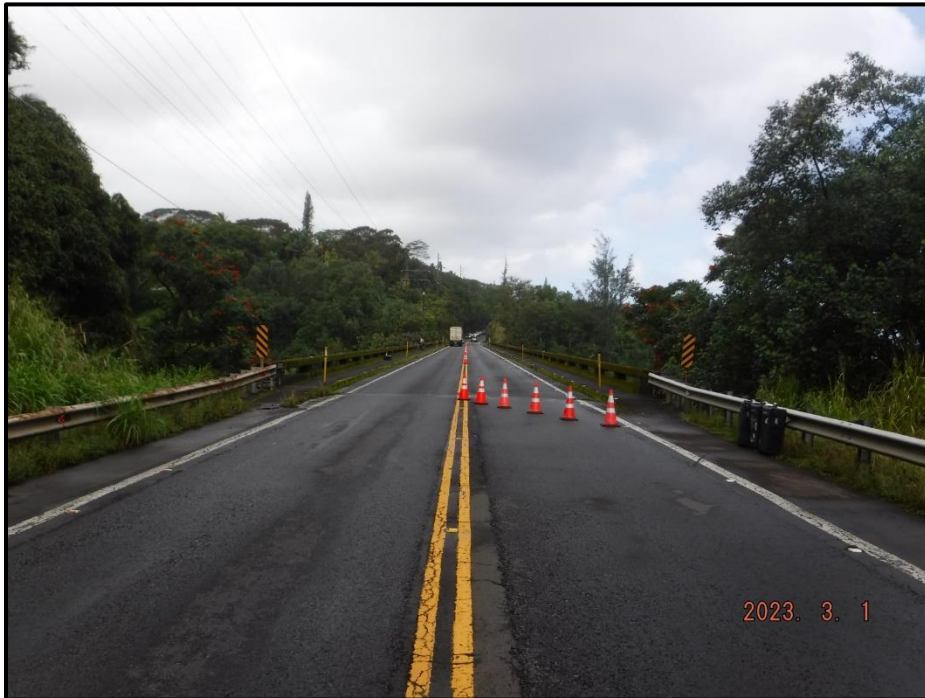
Photograph 3. South approach, looking north.
