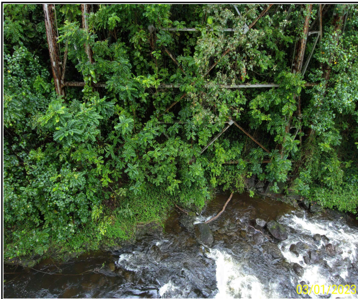
Photo 7. North embankment and channel alignment, looking north
