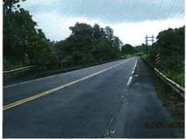
Nanue Bridge approach looking north
