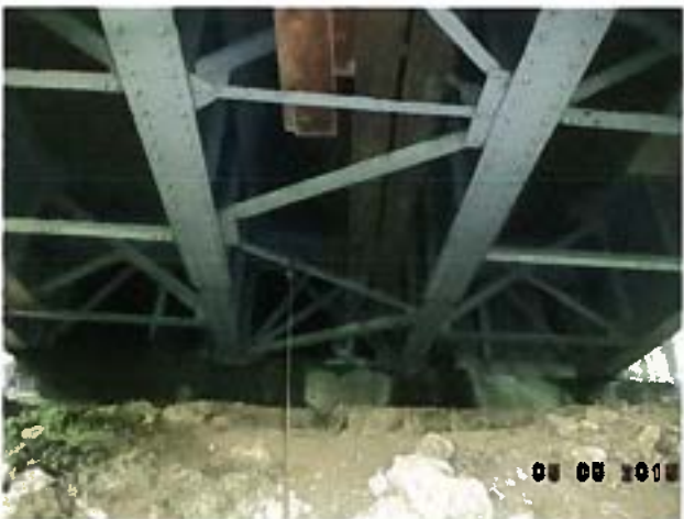
Nanue Bridge north abutment
