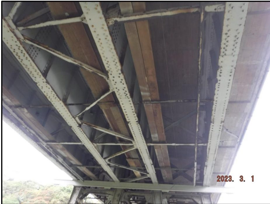
Photograph 9. Typical superstructure (Span 4 shown), looking north.
