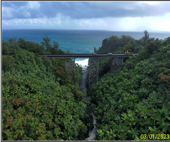
Photo 1. Upstream (west) elevation, looking east
