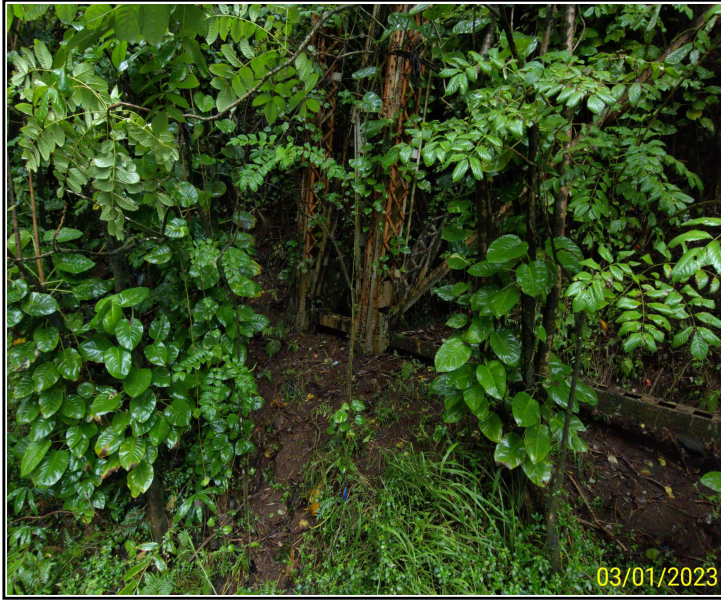
Photo 17. Bent 6, Columns C and D, looking north
