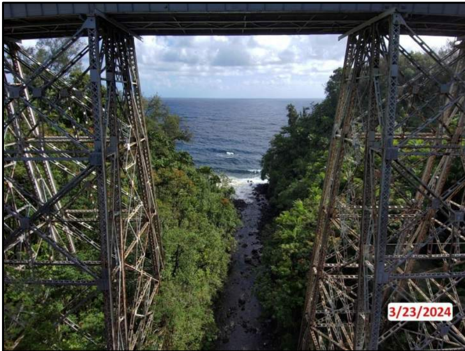
Photograph 8. Typical towers (Bents 5 and 6 at Towers 3 and 4 shown, respectively), looking east.
