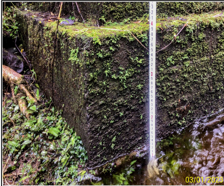
Photo 9. Bent 5, Column A footing, looking south. Exposure, up to 4' H
