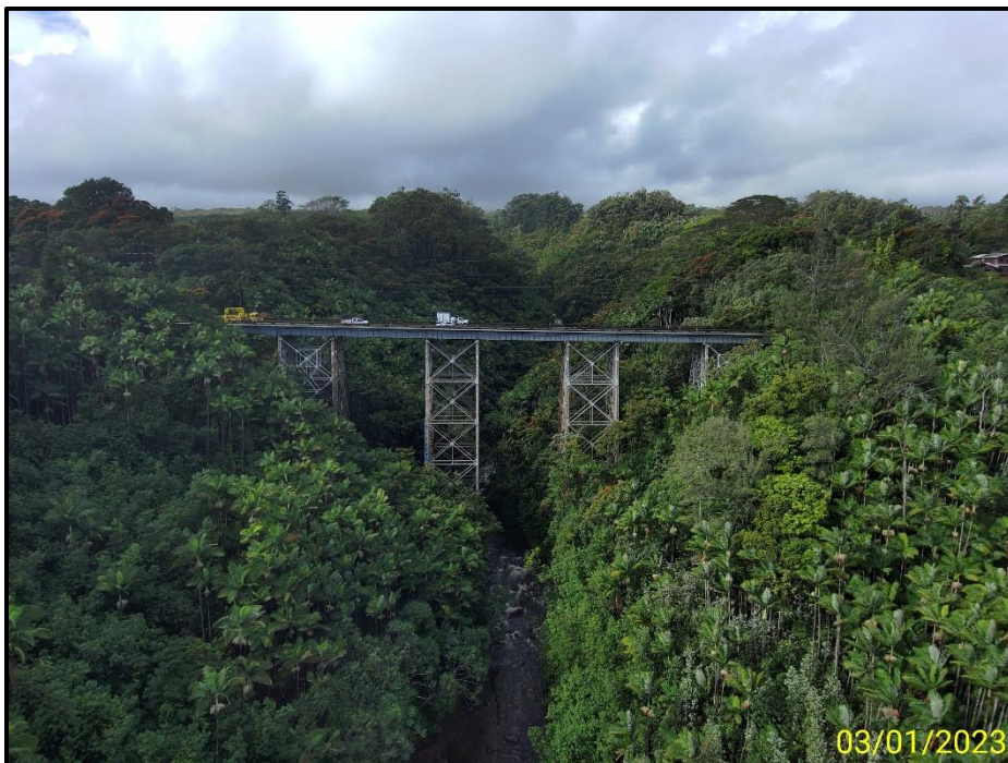
Photograph 2. East (downstream) elevation, looking west.
