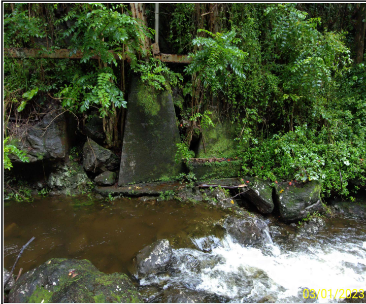
Photo 13. Bent 6, Columns A and B, looking north
