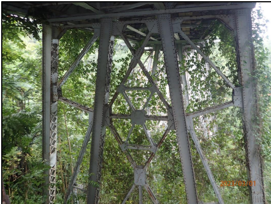
Photograph 12. Bent 1 at Tower 1 (south face shown), looking north.
