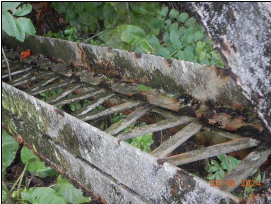
Photograph 112. Tower 4, Level 5, Column C, mid-diagonal mid-length, interior top angle, looking north. 100% section loss for most of length of horizontal flange. Approximately 20% loss of cross sectional area, CS3.
