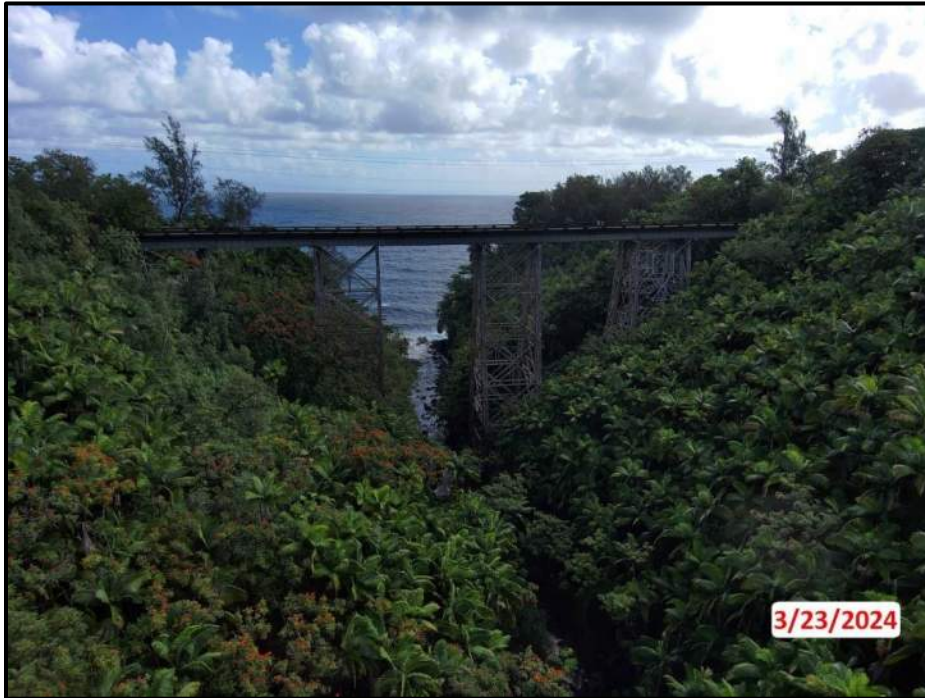
Photograph 2. West (upstream) elevation, looking east.
