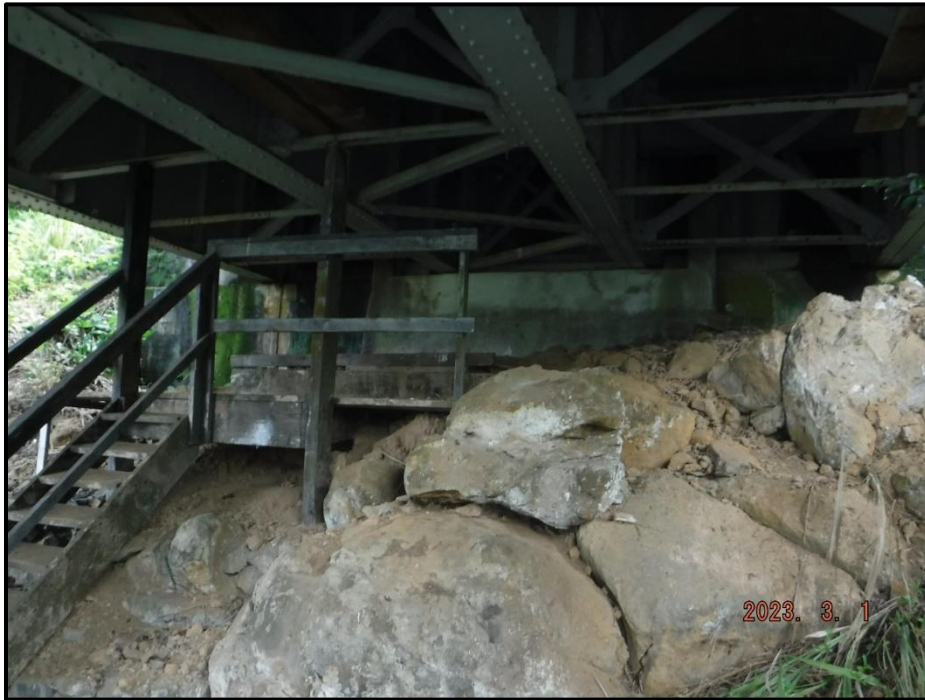
Photograph 11. South Abutment, looking south.
