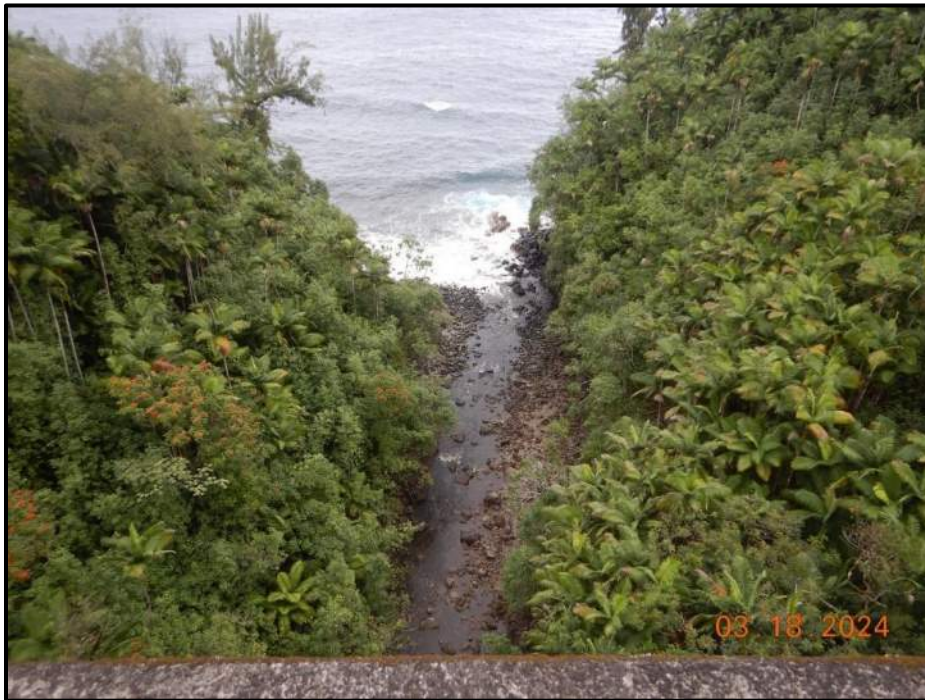
Photograph 6. Downstream channel, looking east.
