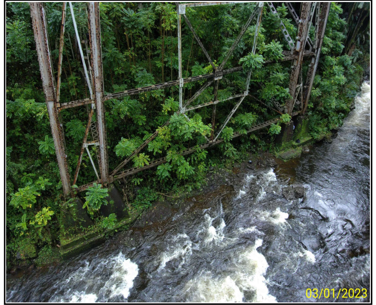
Photo 6. South embankment and channel alignment, looking south
