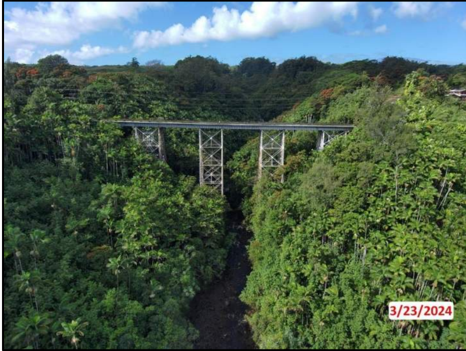
Photograph 1. East (downstream) elevation, looking west.
