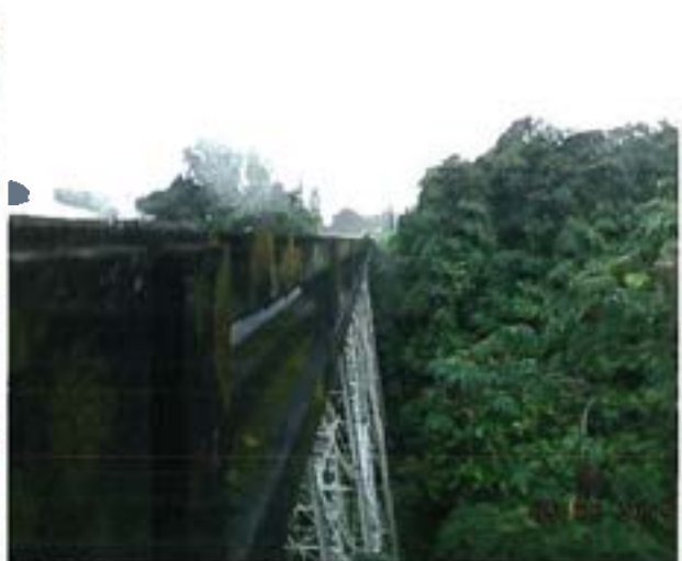
Inlet end of Nanue Bridge.
