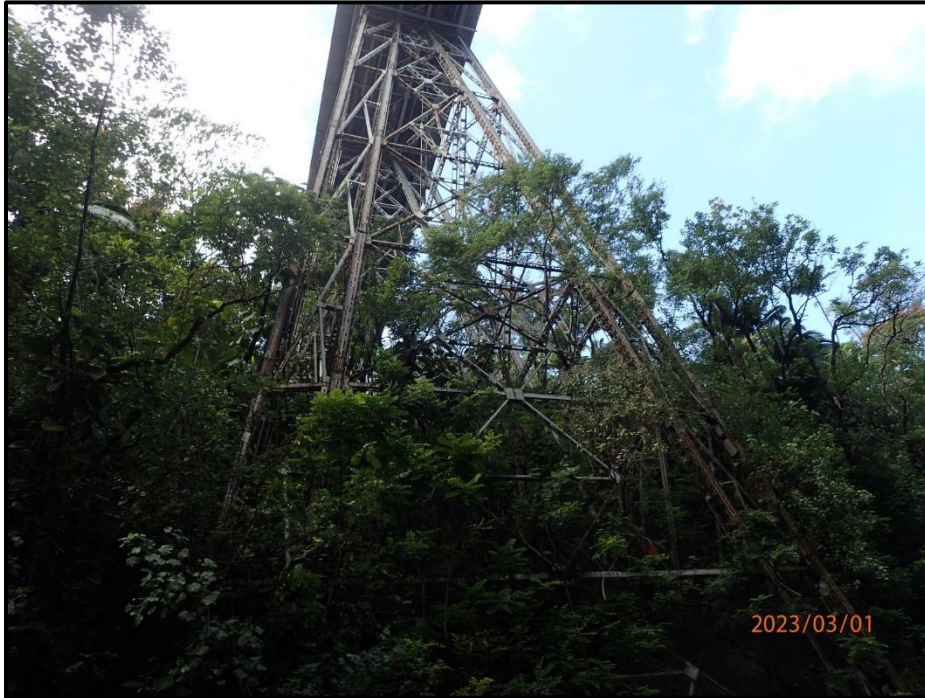
Photograph 13. Bent 6 at Tower 4 (south face shown), looking north.
