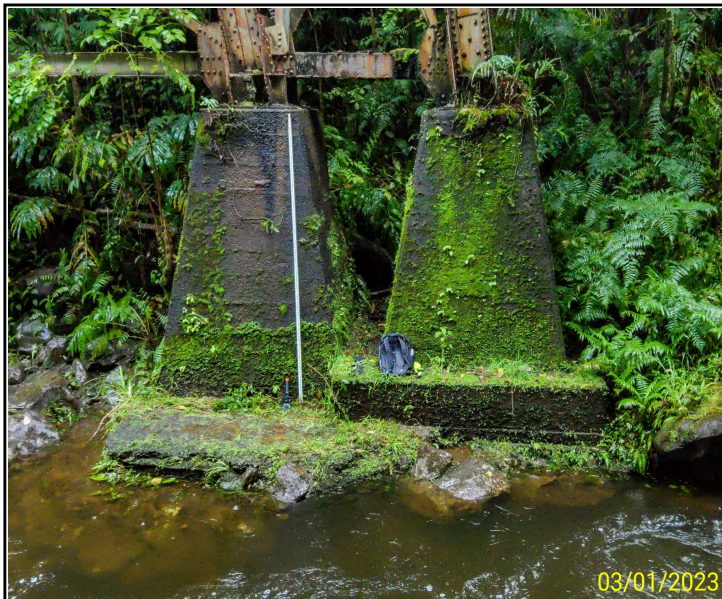
Photo 11. Bent 5, Columns C and D, looking south
