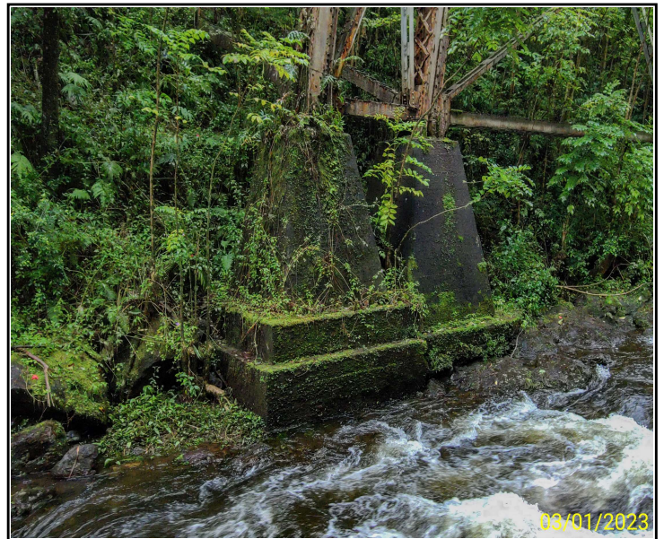
Photo 8. Bent 5, Columns C and D, looking south
