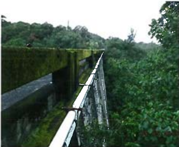
Outlet end of Nanue Bridge.
