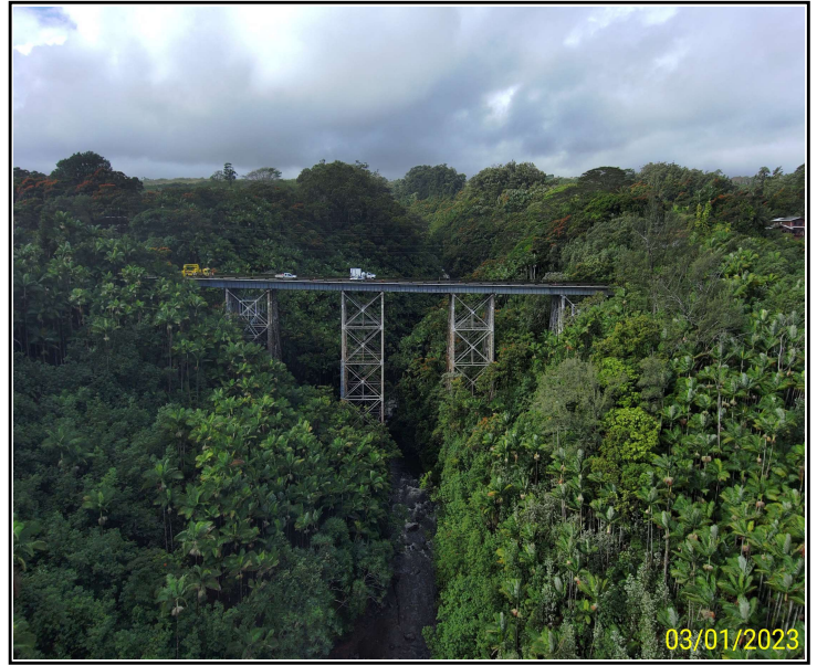
Photo 2. Downstream (east) elevation, looking west
