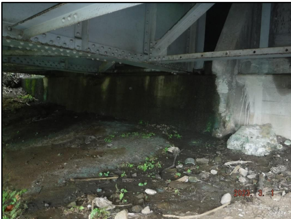
Photograph 10. North Abutment, looking north.
