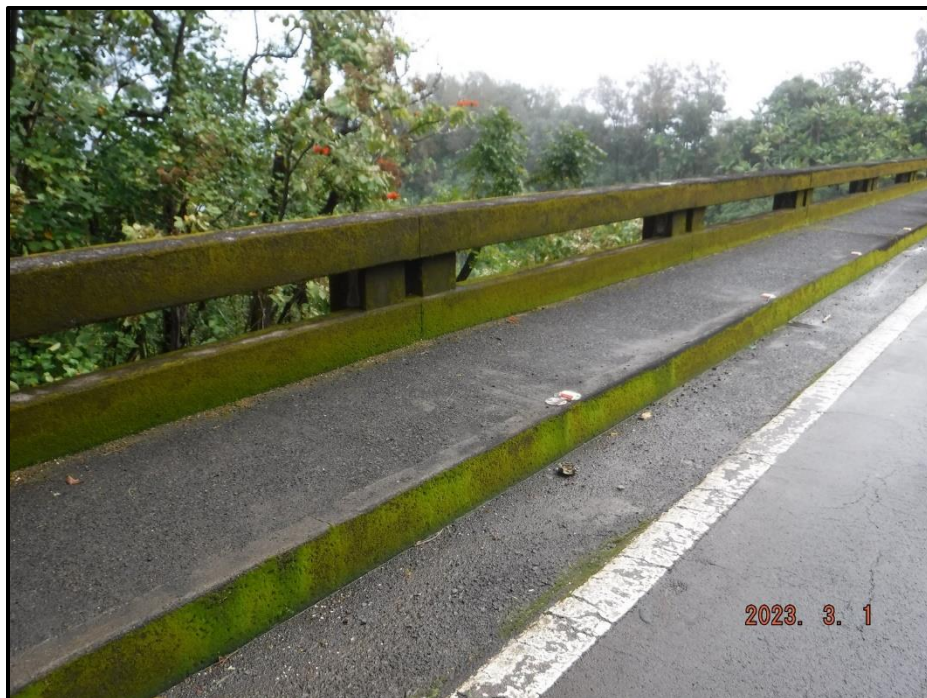
Photograph 8. Typical bridge railing (east railing shown), looking southeast.
