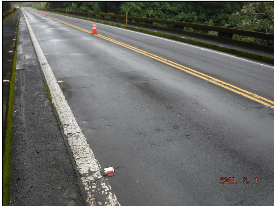
Photograph 7. Top of deck/wearing surface (Spans 8 to 9 shown), looking southwest.
